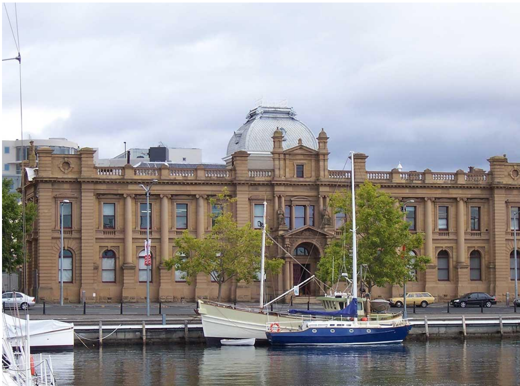
1815 onwards - Customs House and Bond Store, 19-21 Davey Street, Cnr Dunn Street, Hobart, Tas
